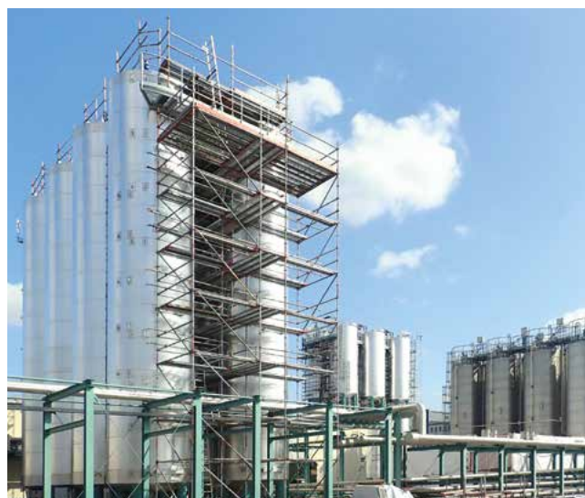
In the foreground: All eight blending tanks have been erected. Until the blending of the first batch in October 2019 pipelines and electro-technics have to be installed yet
