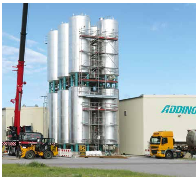
Last construction stage: Installation of pipelines leading to the central register
