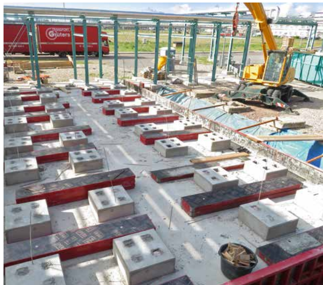
First construction stage: Foundation for the eight new blending tanks
