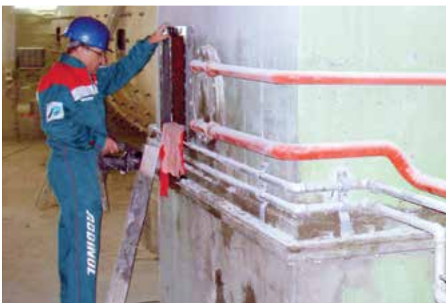
At the recommendation of Mr. Haak, the inspection cover at the Wittekind cement works was first expanded into an opening in the upper section of the housing, in order to enable entry into the inside of the gear unit and thus be able to inspect the gears up close.
